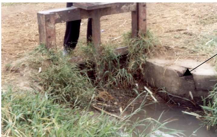
Figure 14: Doho rice scheme damaged water control structure
