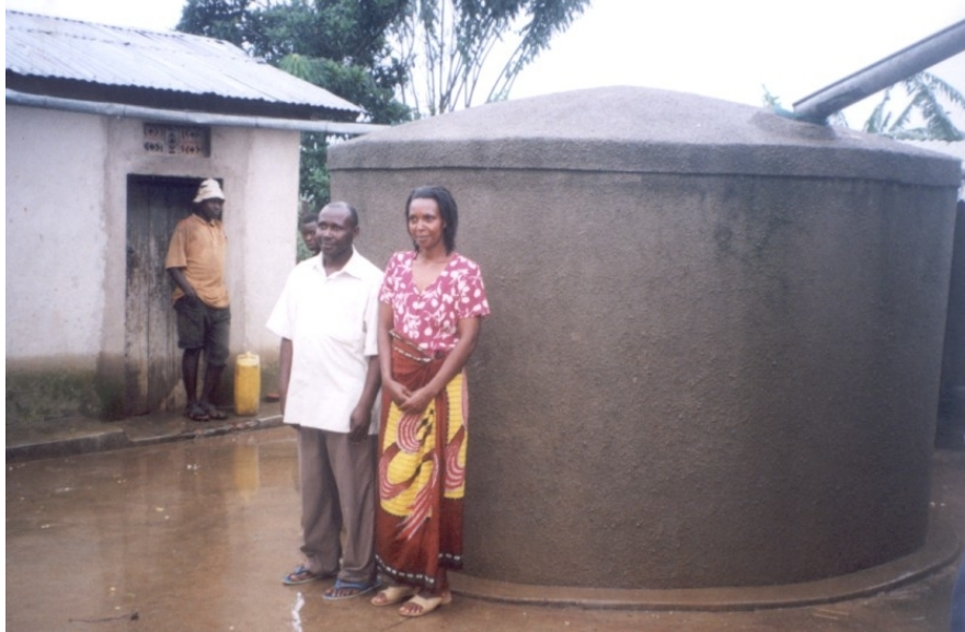
Figure 4: Ferro Cement tank (12 m 3 ) for Mr. Kanyarutokye Edward
