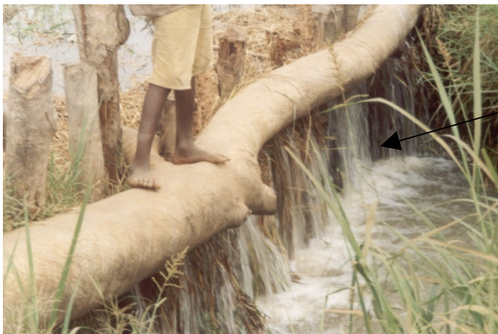
Figure 13: Doho rice scheme poor water control structure
