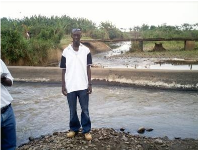
Figure 10 Déviation Barrage and de-siltation system (Bugarama)
