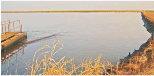
Figure 6.4: Experimental reed bed for the treatment of oil wastewater at Heglig (Source: HCENR, 2007)
