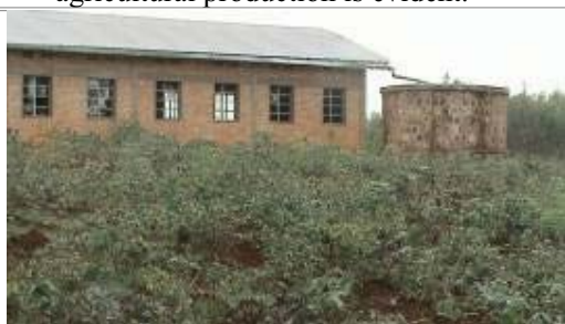
Figure 24 : Collecting rainwater for domestic consumption at GASORWE (MUYINGA)
