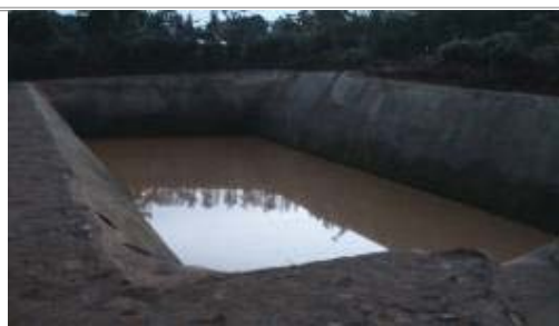
Figure 25 : Collecting rainwater for irrigation at BUGABIRA (KIRUNDO)
