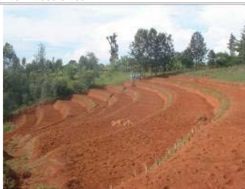
Figure 27 : View of a radical terrace recently constructed at GITEGA
