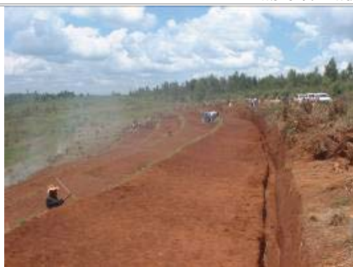
Figure 26 : Construction of a radical terrace in KARUZI province
