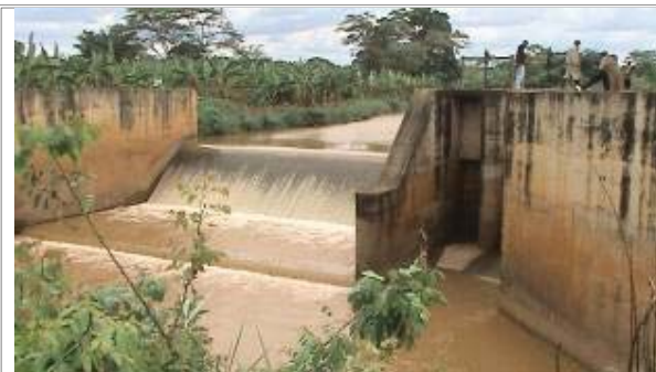
Figure 20 : View of the spillway-dam on the Mutsindozi river (SUCOMO)
