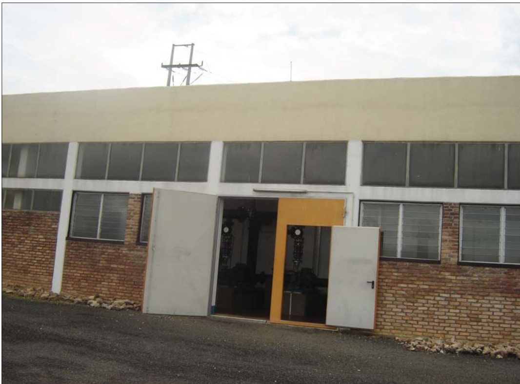
PHOTO 9.14: Water extraction and treatment at Mirambi in Ngenda
