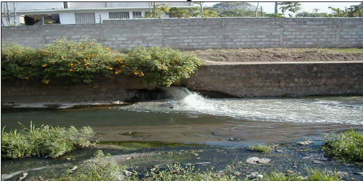
Figure 02: Raw municipal effluent discharging into the Mirongo River (in Mwanza) before closure of the by-pass
