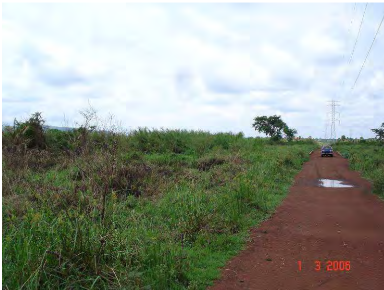
Photo 2. Existing TL between Tororo and Malaba, Uganda
