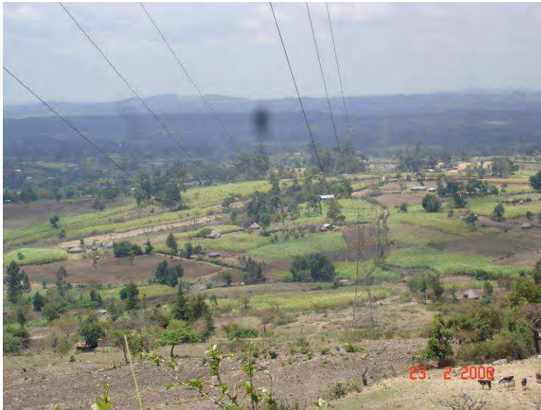
Photo 1. Existing transmission line, Nandi escarpment near Kabiyet
