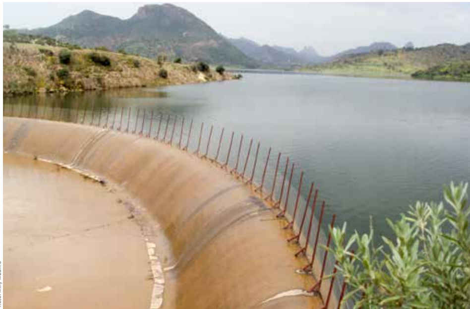
Storage dam in Ethiopia
