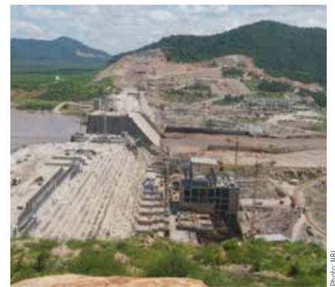
GERD dam under construction
