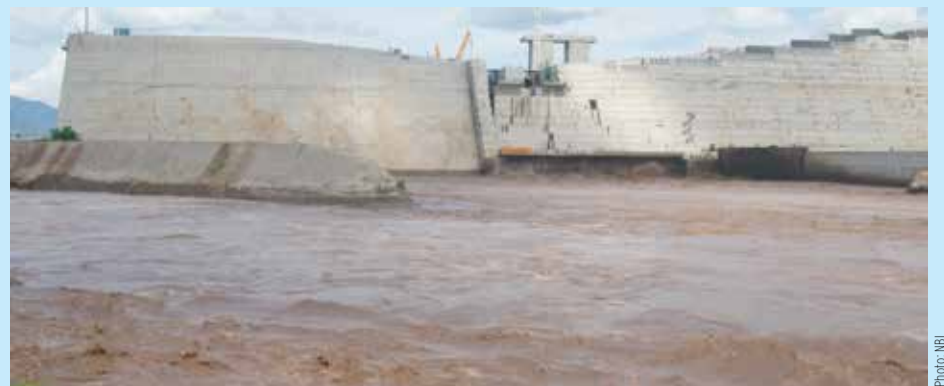
GERD dam under construction
