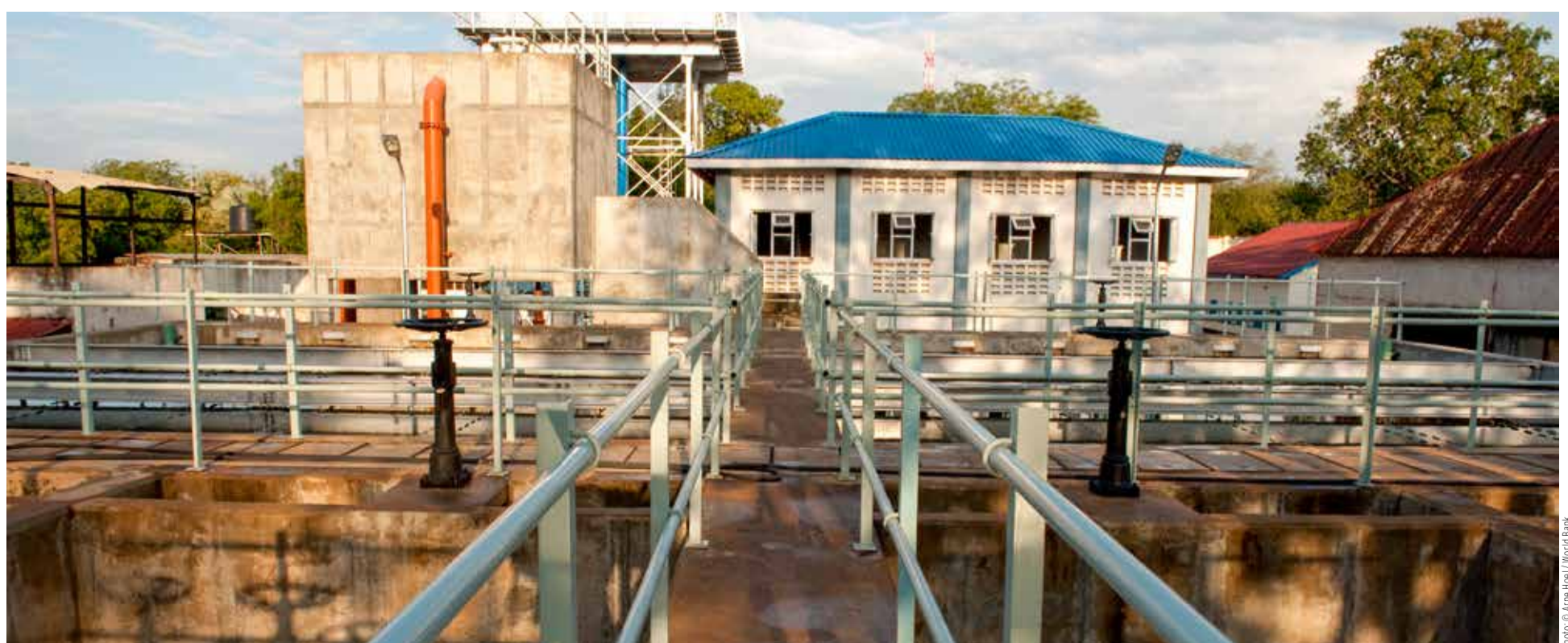
The renovated water treatment plant in Juba, South Sudan
