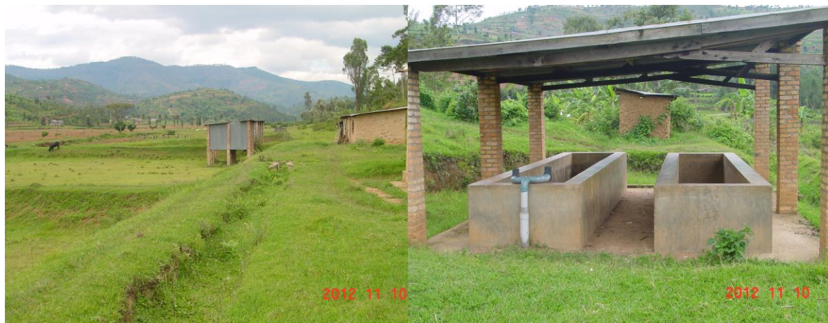
Plate 6-34: Fish ponds of the old Aquaculture Project & Fish fry aeration and preparation chambers
