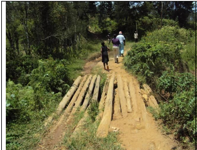
Plate 6-9: Temporary Bridge to the project area
