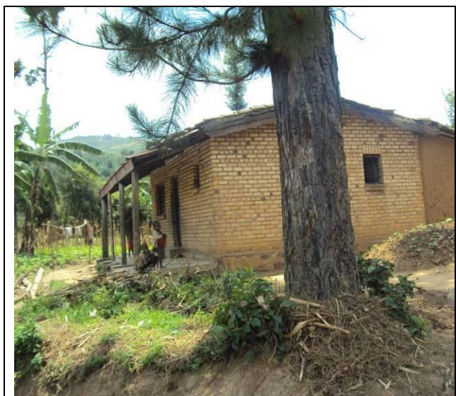
Plate 6-1: A structure in the Project Area
