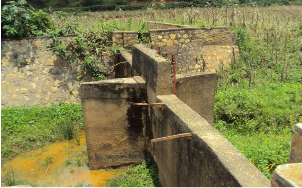
Plate 6-13: Water Infrastructure in the Project Area
