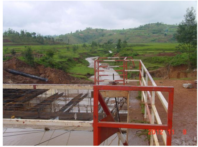
Plate 6-32: KfW project; dam and weir supplying 178Ha Plate 6-33: Second weir being built by KfW a few kms upstream of dam downstream of river Mwogo
