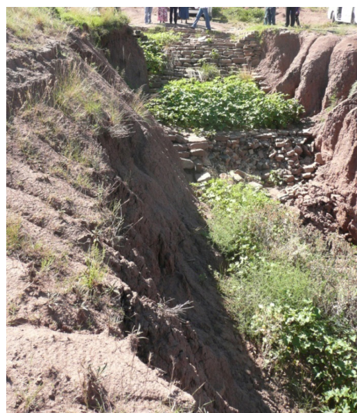
(b) Gully controlled with stone check dam (photo by B. Mati)
