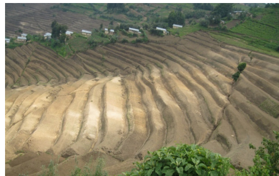
Figure 3.11 (a) Sketch of reverse slope bench terrace (b) Newly constructed reverse slope bench terrace (photo courtesy of J.J. Mubinda)
