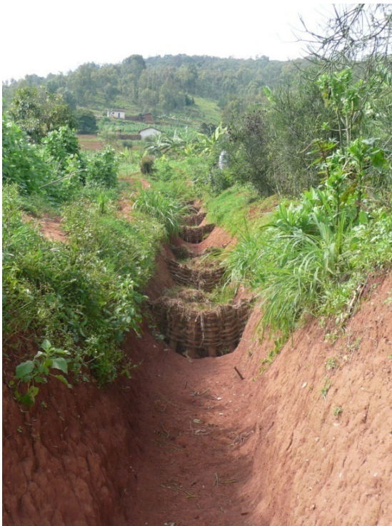
Figure 4.2 (a) Artificial waterway with scour checks ( photo by B. Mati ) (b) Grassed Artificial waterway ( photo courtesy of J.J. Muhinda )
