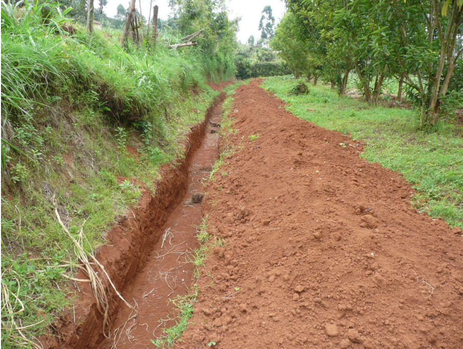
Figure 2.1 A newly excavated diversion ditch (photo by B. Mati)
