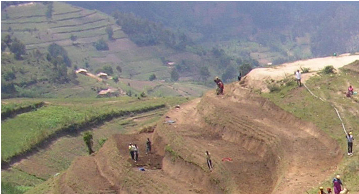
Figure 3.1 Terraces reduce slope steepness and slope length (photo by J. Gassasira)
