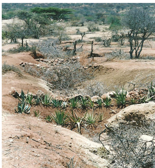
Figure 5.9 (a) Sisal used to rehabilitate gully controlled with stone check dams (b) Grass cover for rehabilitated gully (photos by B. Mati)
