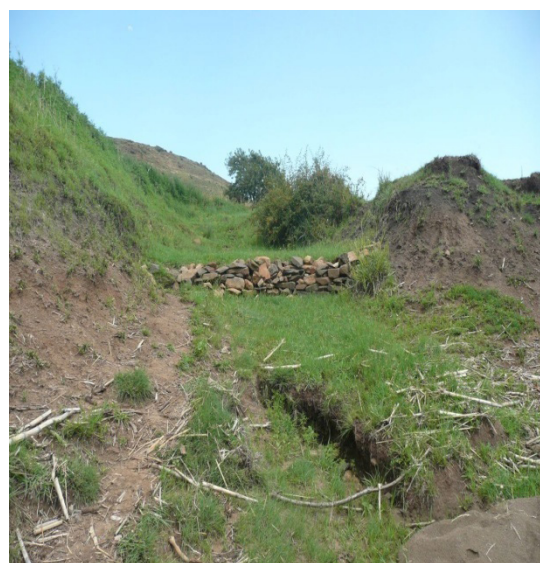
Figure 5.9 (a) Sisal used to rehabilitate gully controlled with stone check dams (b) Grass cover for rehabilitated gully (photos by B. Mati)
