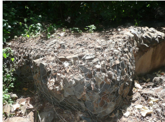
(b) Gabion box filled with stones for gully control (photo by B. Mati)
