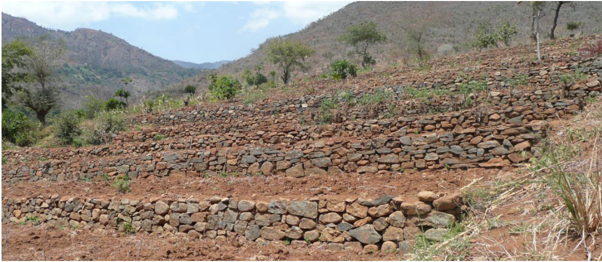
Figure 3.5 Stone lines laid on the contour to create terraces (photo by B. Mati)
