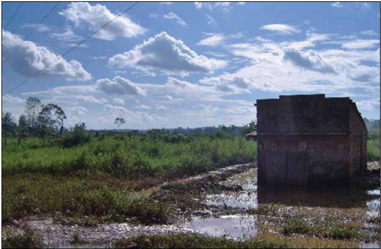
Photograph 10: Effects of unplanned settlements on a wetland include flooding and submergence of buildings - Photo by Joseph Oonyu
