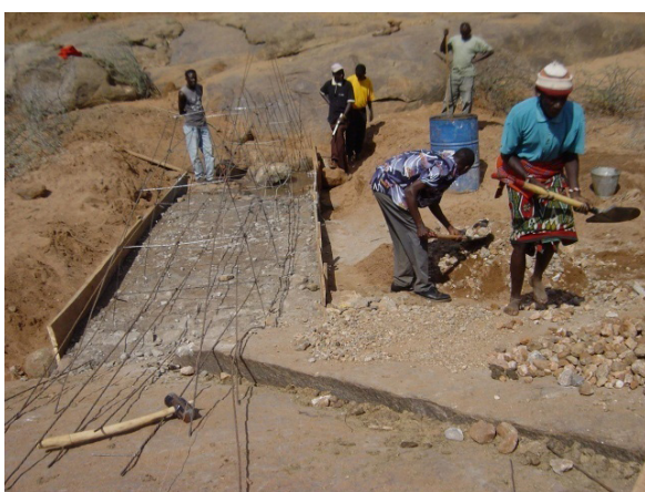
Figure 5.5 (a) Sand dam under construction (photos by Nancy Mati) (b) Sand dam with gravity outlet to storage tank
