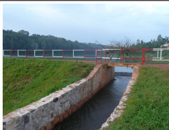
(b) Diversion chute from an earth dam
