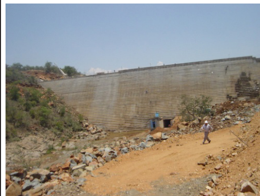
(b) Earth dam construction near completion – front is lined with masonry
