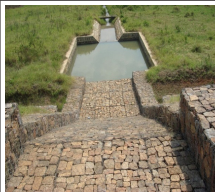
(b) The completed spillway of a dam (photo by B. Mati)
