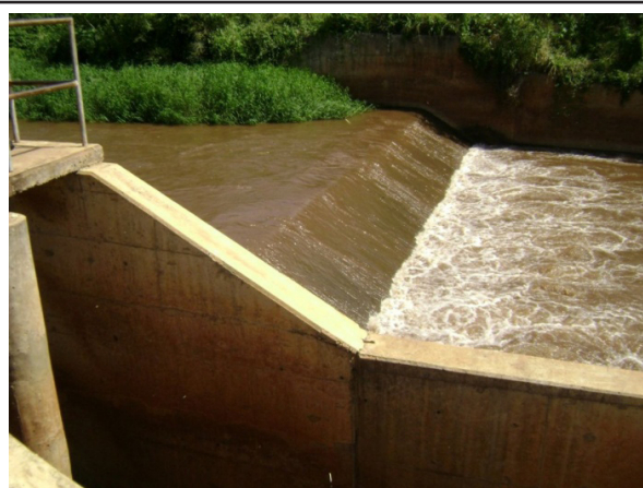
Figure 2.3 Water diversion from small earth dam using a weir (photos by B. Mati)
