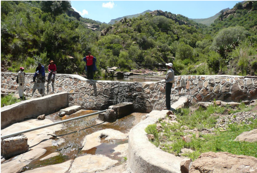
Figure 3.7 Weir located below rocky hills for RWH with piped water supplies (photo by Nancy Mati)
