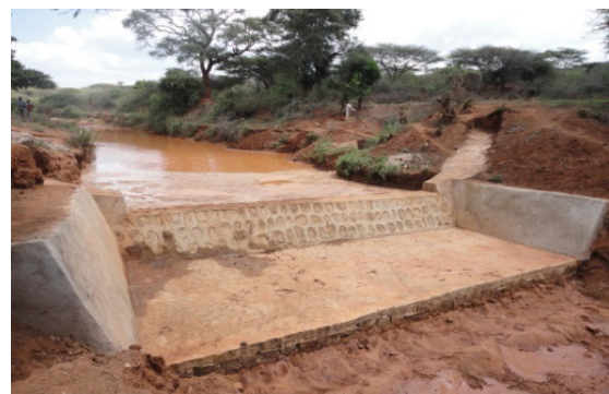
(b) A sand dam showing apron (source Alemu Seifu, 2011)
