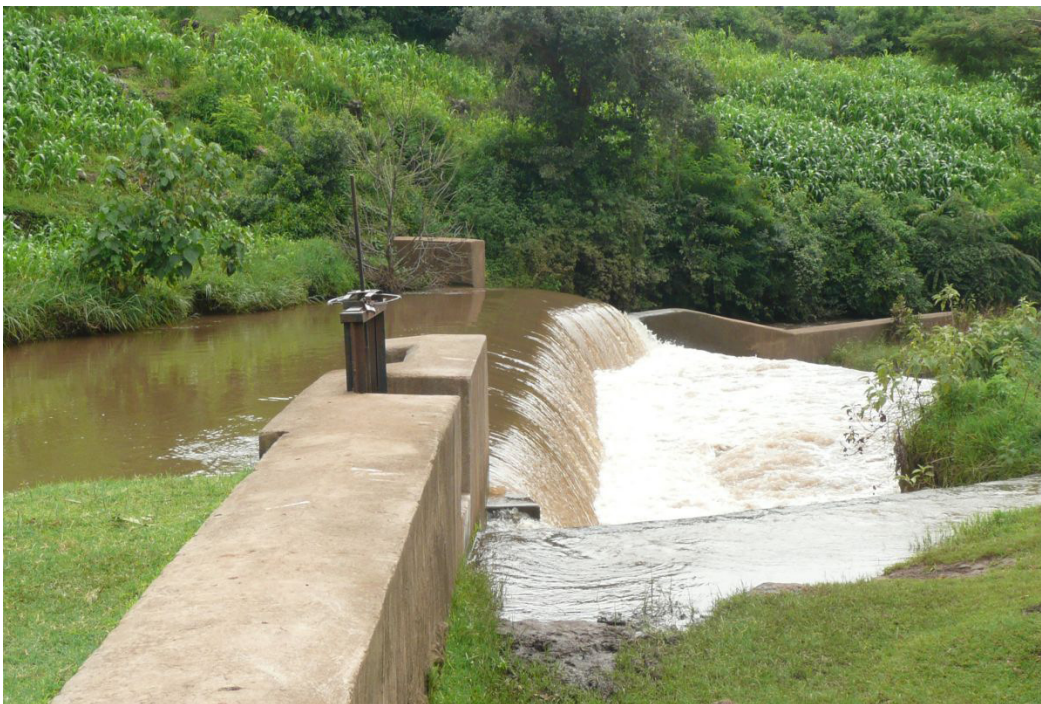
Figure 3.1 Typical weir for flood water harvesting and stream diversion (photo by B. Mati)
