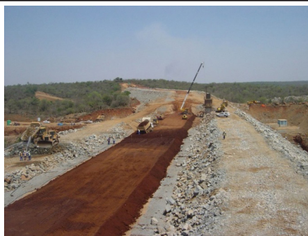
Figure 2.10 (a) Earth-fill dam under construction (photos by Nancy Mati)
