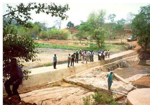
Figure 5.5 (a) Sand dam under construction (photos by Nancy Mati) (b) Sand dam with gravity outlet to storage tank
