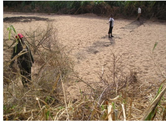
(b) Subsurface dam just after construction
