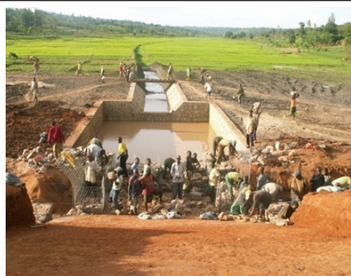
Figure 2.9 (a) Spillway under construction (photo by Jean Muhinda)
