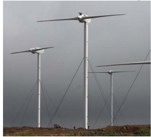
Wind farm under construction at Ashegoda, near Mekelle, Ethiopia.
