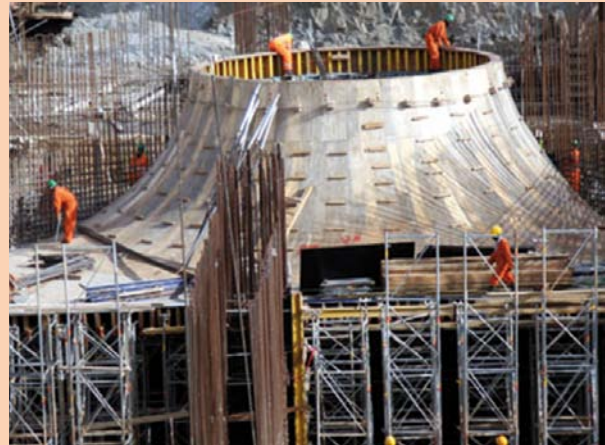
Bujagali power plant under construction.
