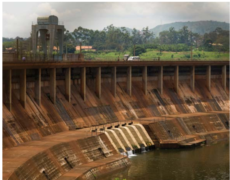
Nalubaale Hydroelectric Power Station (Owen Falls Dam), Uganda.
