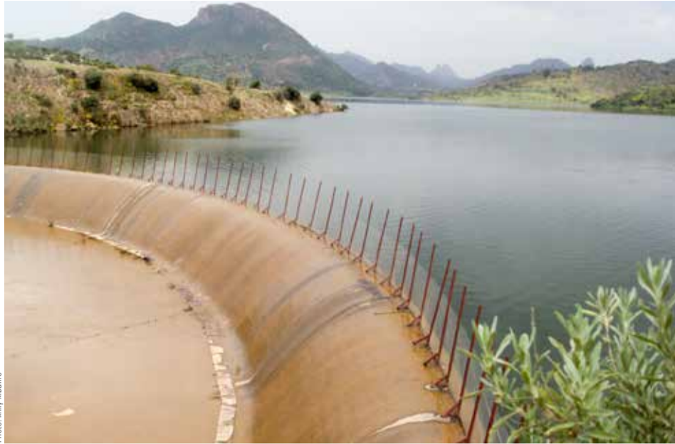
Storage dam in Ethiopia
