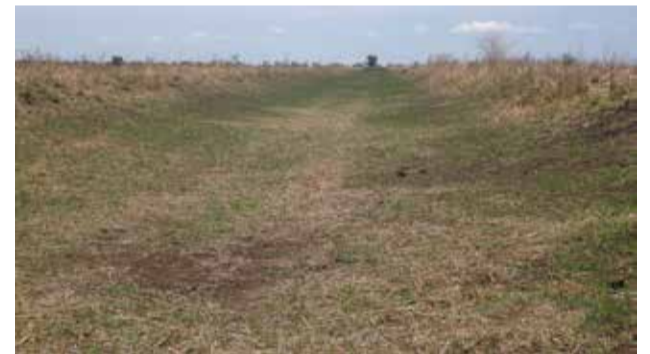
Secondary canal in Aweil rice scheme during dry season
