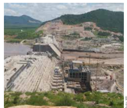
GERD dam under construction
