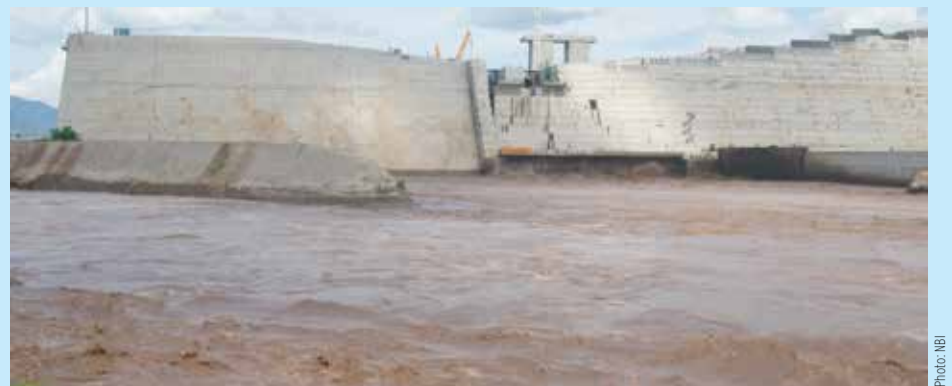
GERD dam under construction
