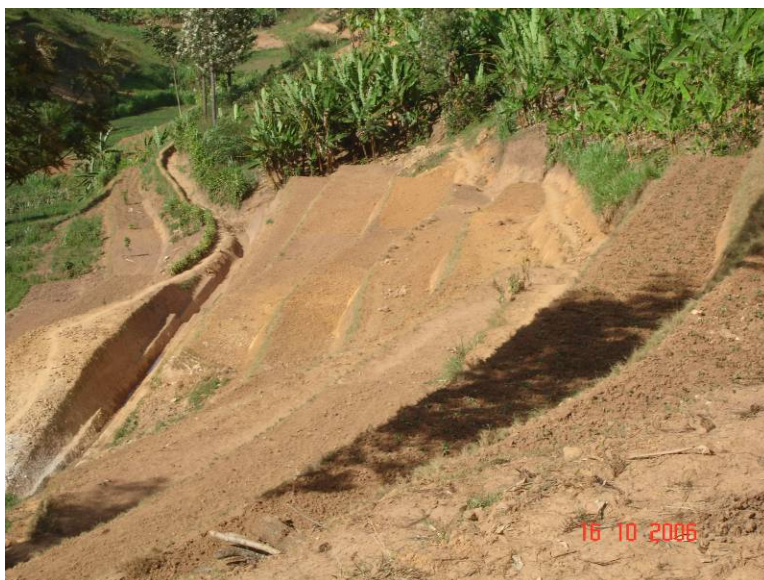
SOCAMAF demonstrates construction of a hillside irrigation canal & radical terraces
