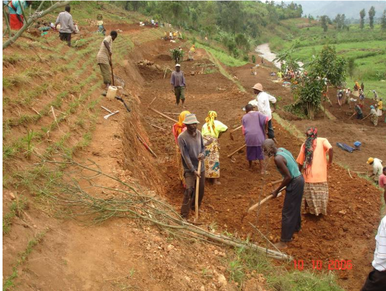
Community members in the sectors of Rwaza and Muko being trained by COOCASTER to prepare radical terraces on the hillside of River Mukungwa
