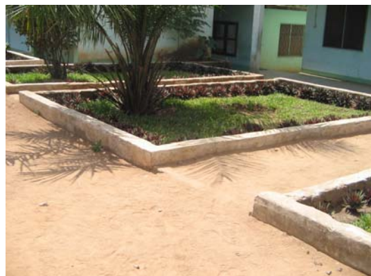
Project to prevent soil erosion at Nganza Secondary School
