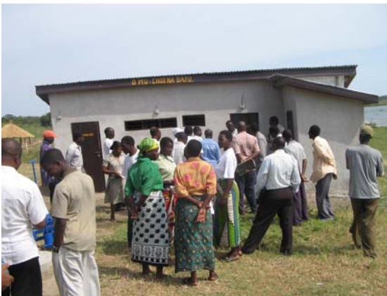
Latrines built by NEP in Ukerewe
