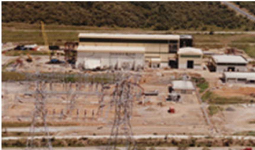
Geothermal power station
