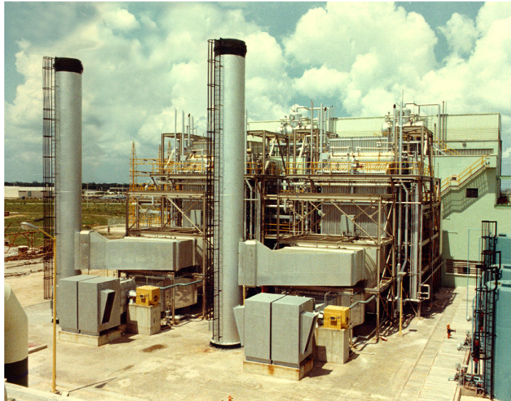
Thermal power station
