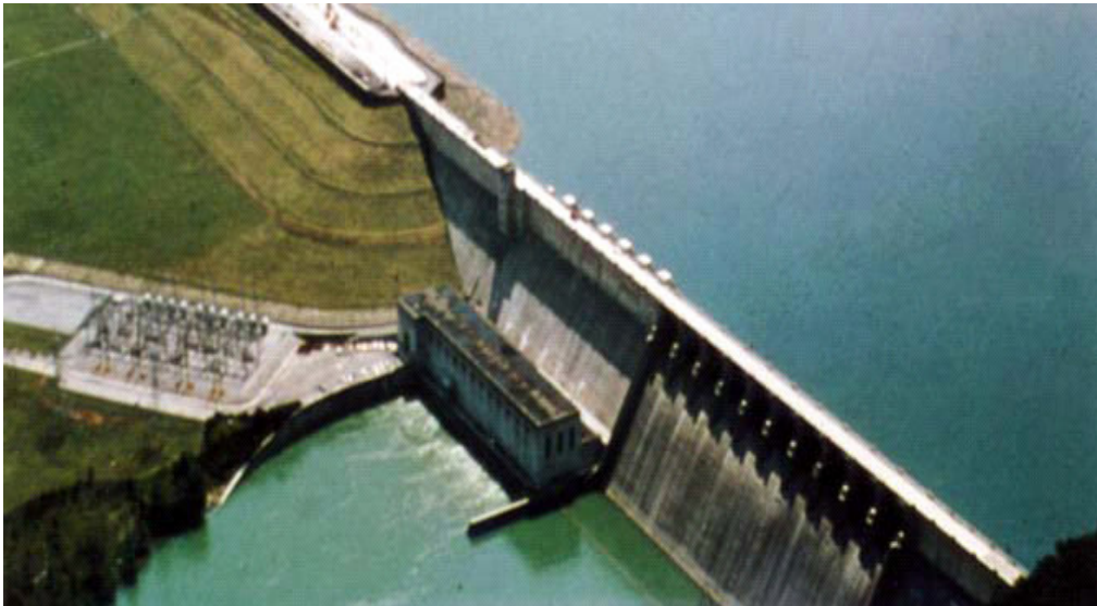
Hydropower dam in concrete
