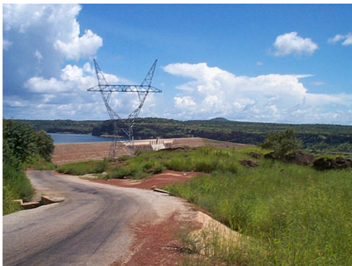
Power transmission line
