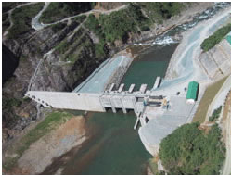
Figure 6.1. The Casecnan dam and multipurpose project
