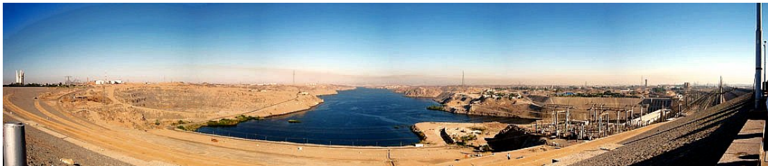
Figure 5.1. Panorama view of High Aswan Dam
