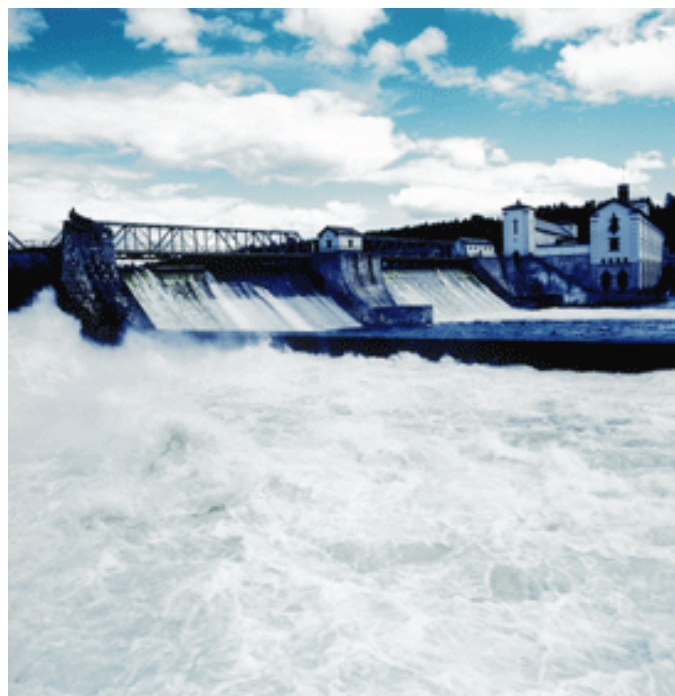
Figure 6.4. Rånåfoss Power Station
