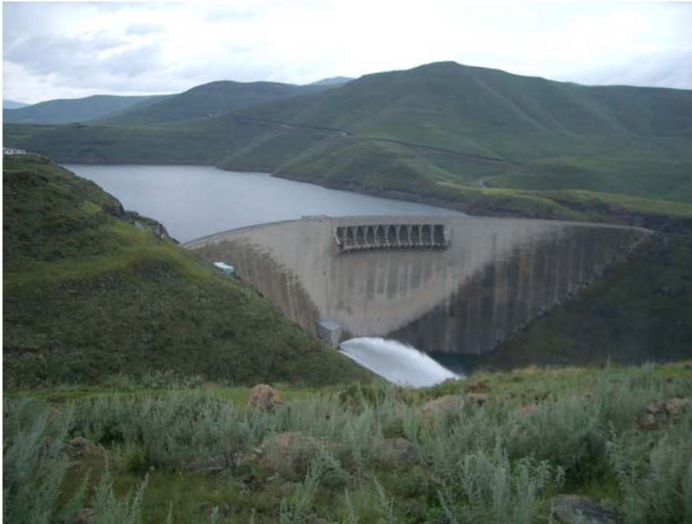
Figure 6.7. The Katse dam in the Lesotho Highlands Water Project
