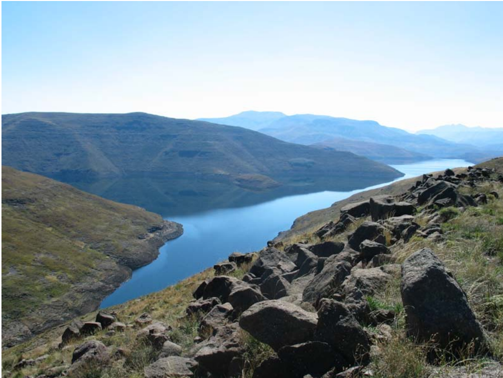
Figure 6.10. Mohale reservoir, Lesotho Highlands Water Project
