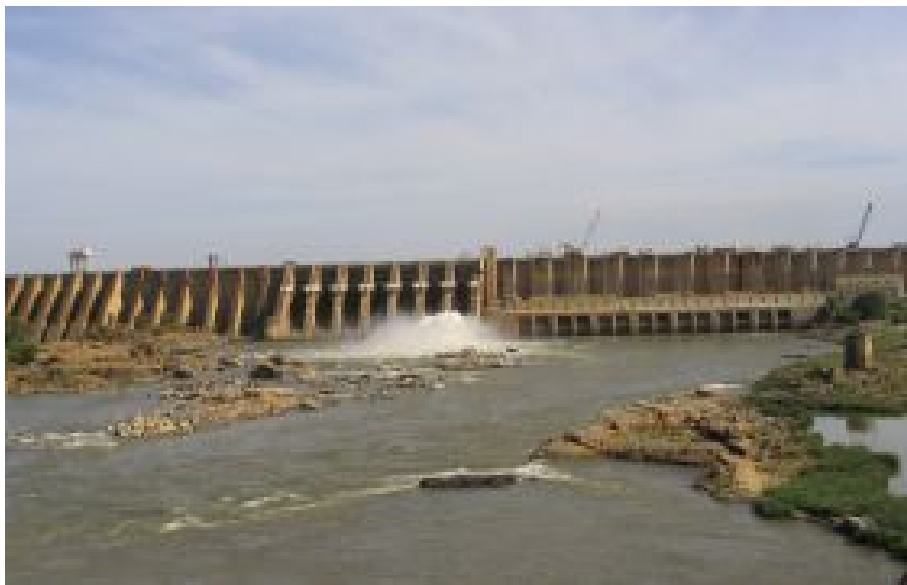
Figure 5.10. The Roseires dam, Sudan
