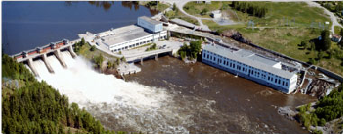
Figure 6.3. One of the many regulation reservoirs, Kykkelsrud Dam and Power Plant
