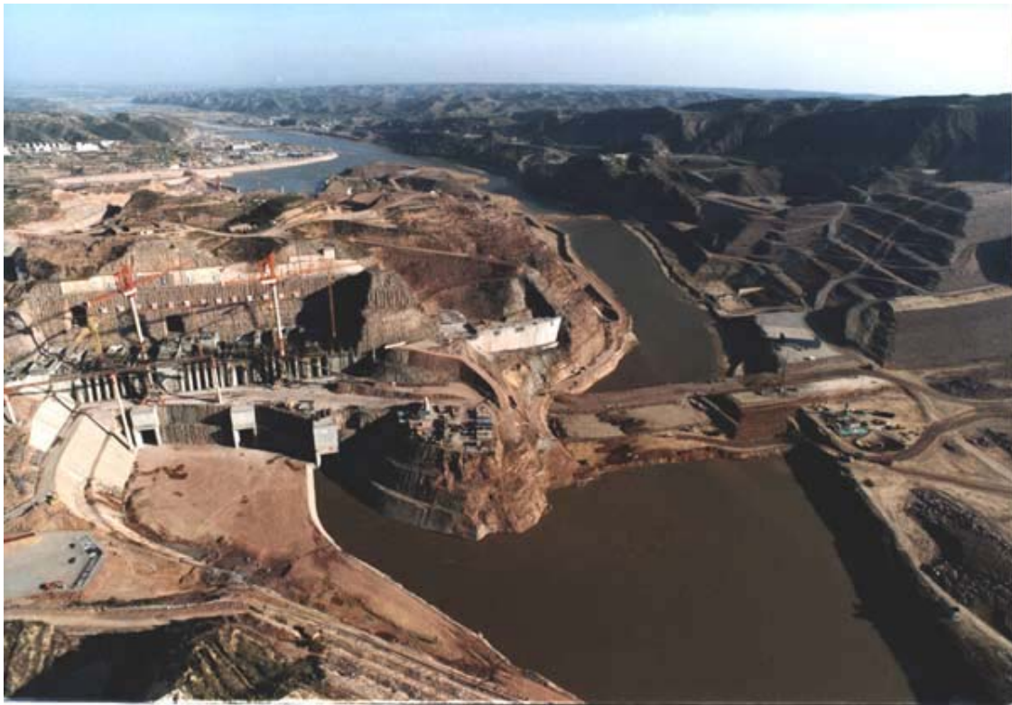
Figure 6.16. The Xiaolangdi dam and intake
