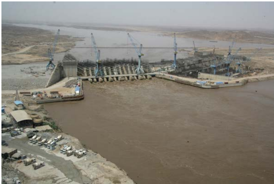
Figure 5.5. Construction of Merwoe dam
