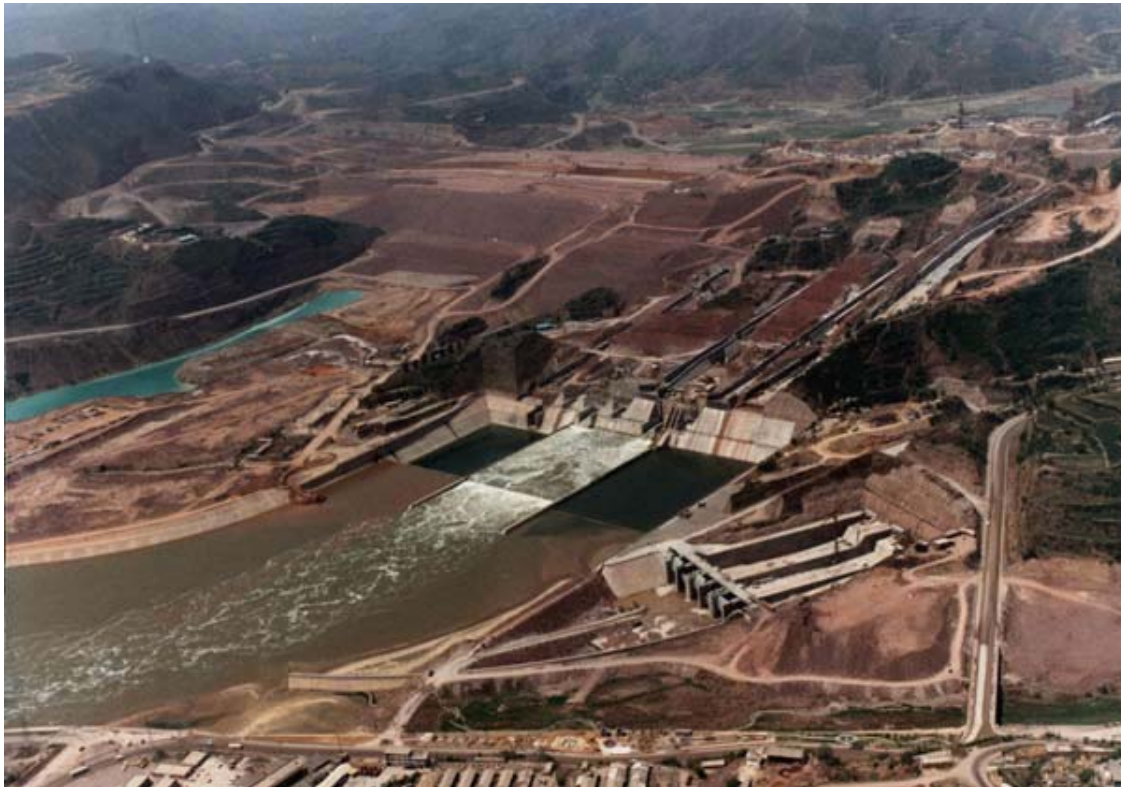
Figure 6.17. Xiaolangdi – Flow discharging through tunnel outlet
