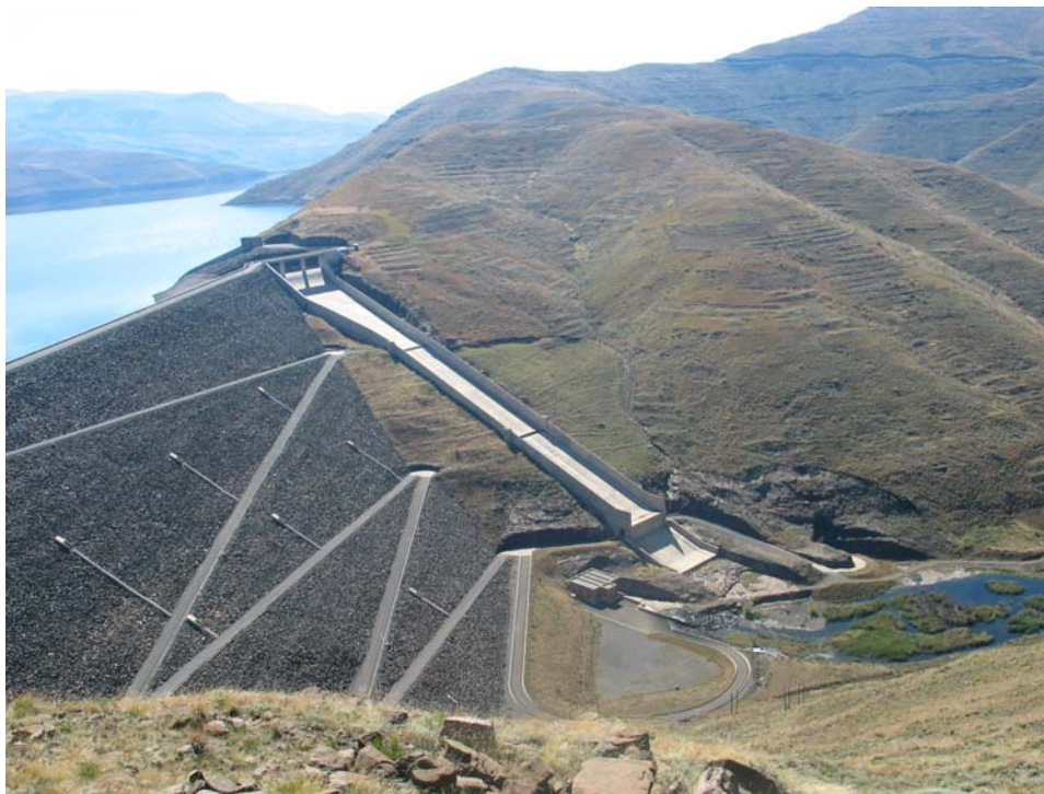
Figure 6.8. Mohale Dam, Lesotho Highlands Water Project
