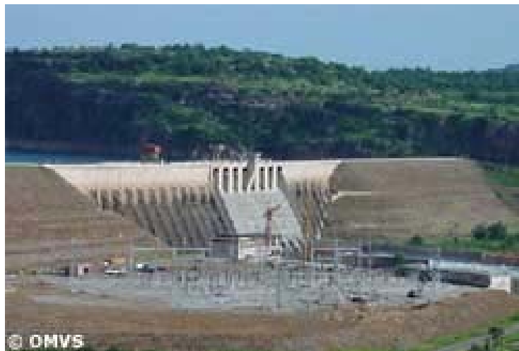
Figure 6.14. The Manantali dam
