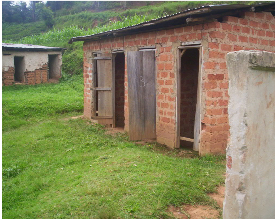
Figure 7 A school's toilet facility
