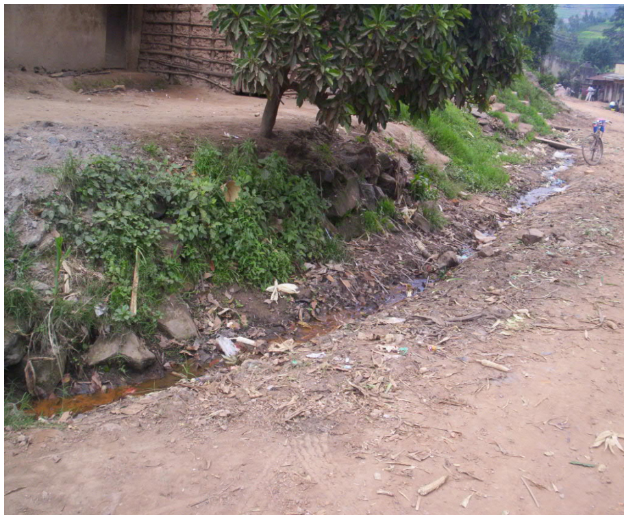
Figure 5 Drainage channel in Katuna
