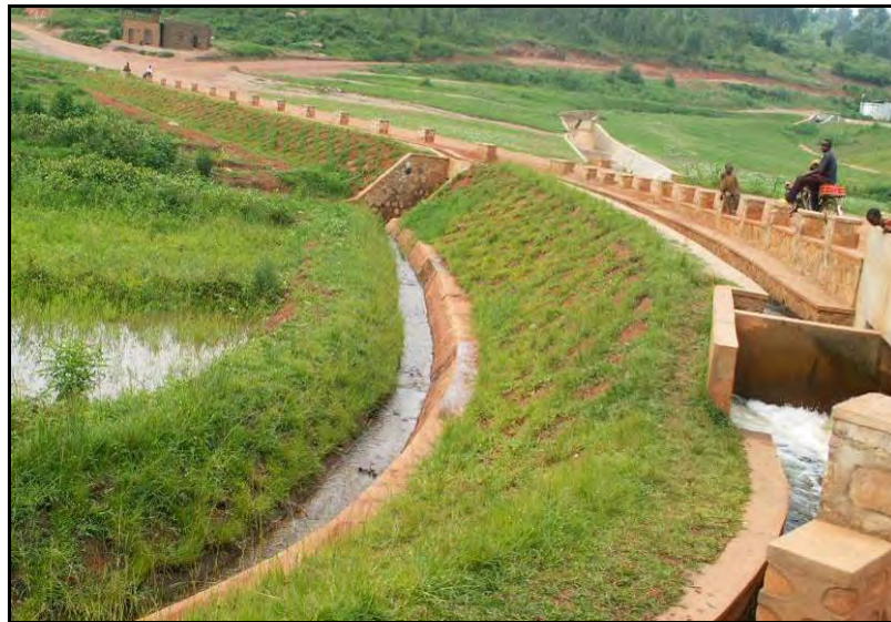
Figure 6.5 - Rwandan marshlands irrigation infrastructure in Kanyonyomba
