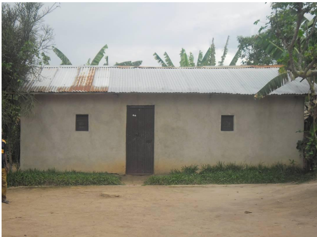
Plate 4.9-8 Iron sheets roofed house structure
