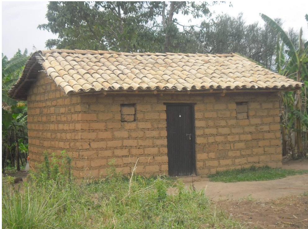
Plate 4.9-7 House structure roofed with local tiles
