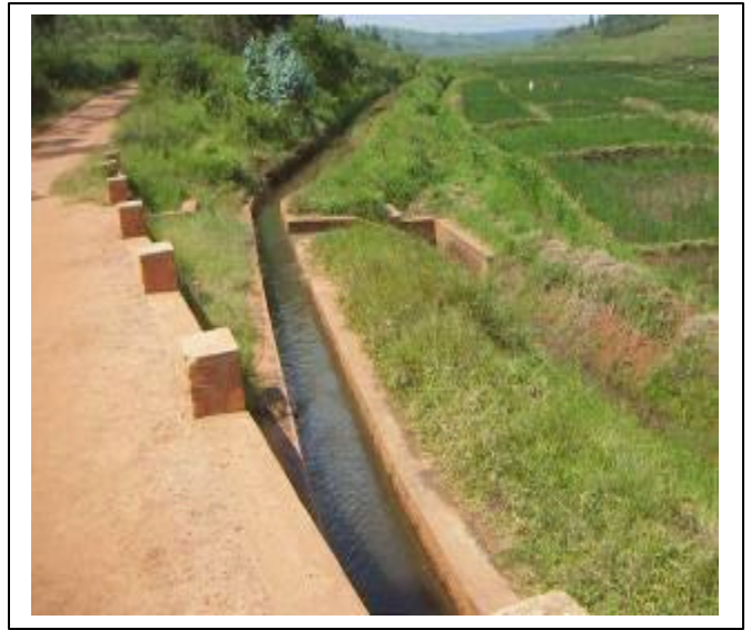
Lined canals contribute to improving efficiency
