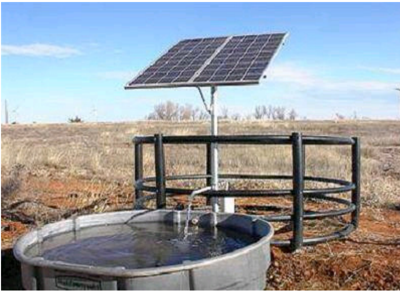
Figure 7.1 A solar powered pump with surface tank (Source: ClimateTechWiki )
