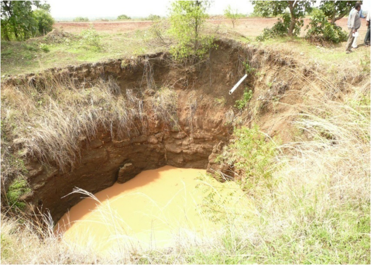
Figure 2.1 (a) Artificial recharge of ground water from road runoff - see inlet pipe (Photo by B. Mati)
