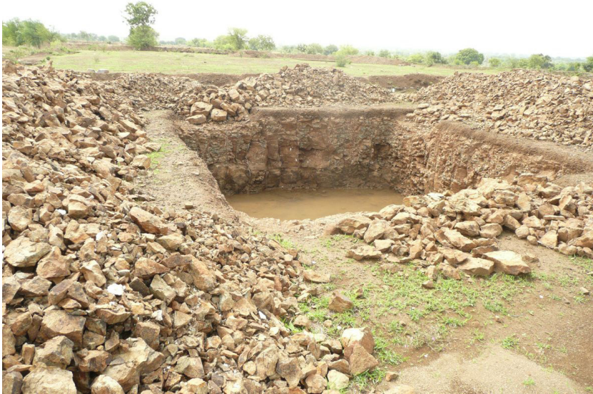
Figure 2.4 Artificial recharge of ground water using percolation pond ( Photo by B. Mati )
