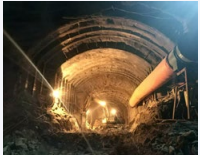
Underground tunnel at the Rusumo project site
