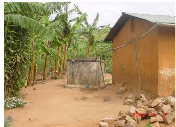
Plate 6-19: Rain water harvesting
