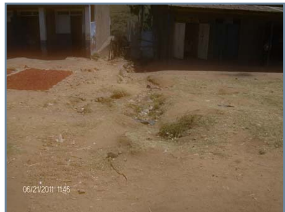
A natural drainage channel directing stormwater to River Lwakhakha from the main road on the Kenyan side
