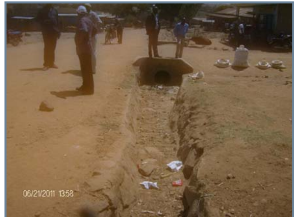
A drainage channel with flexible lining on the Ugandan side
