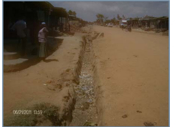
Solid waste swept into the drainage channel from business premises in the background on the Ugandan side
