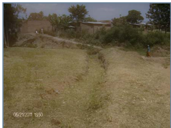
A grassed drainage channel on the Ugandan side
