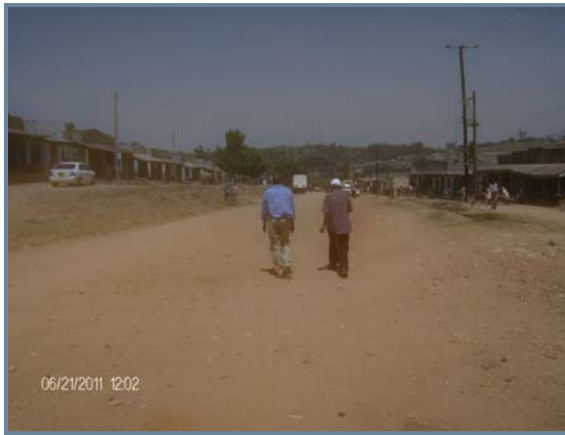
Road surface susceptible to erosion by runoff during storms
