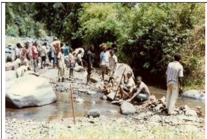
Figure 13.5: Water users gathering at the river intake to their irrigation system to rebuild the intake structure, Kilimanjaro, Tanzania
